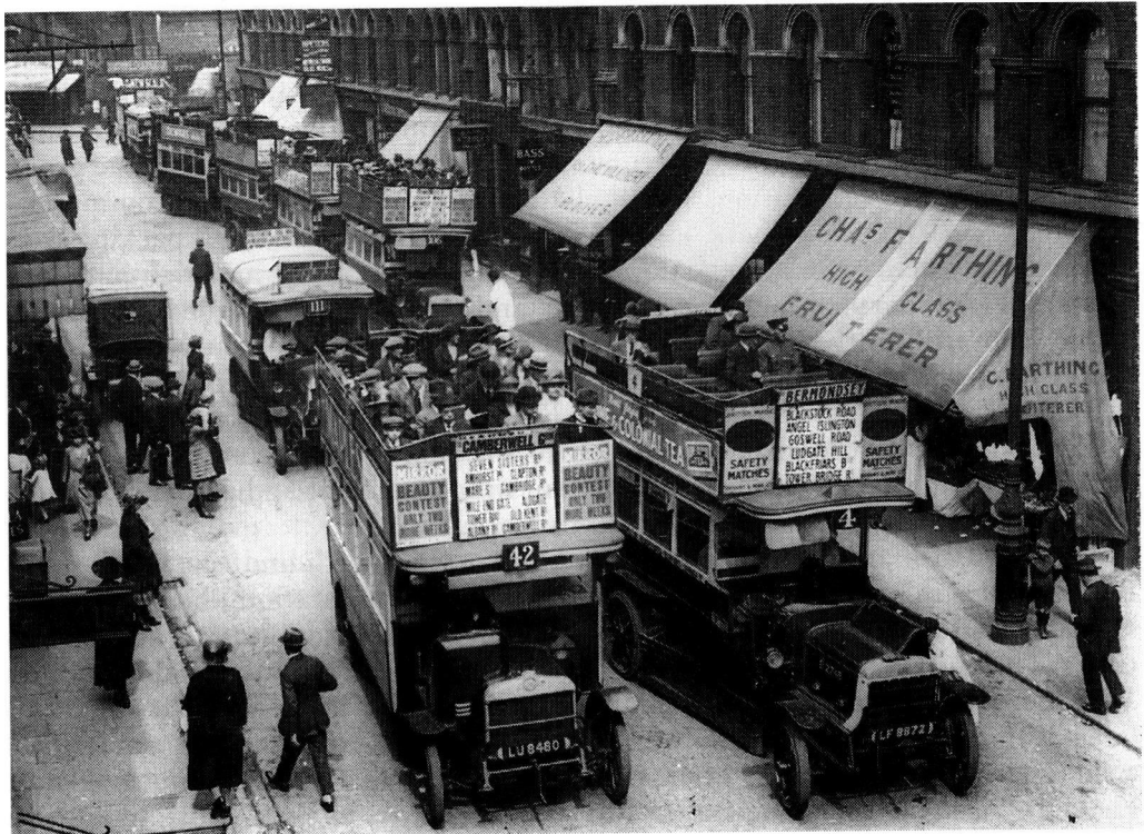
Fig. 10 Station Place in 1923 Copyright London Transport
