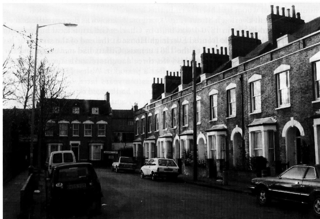
Fig. 7 Everleigh Street, nos. 1-15 (right to left) and no. 17 (detached)
